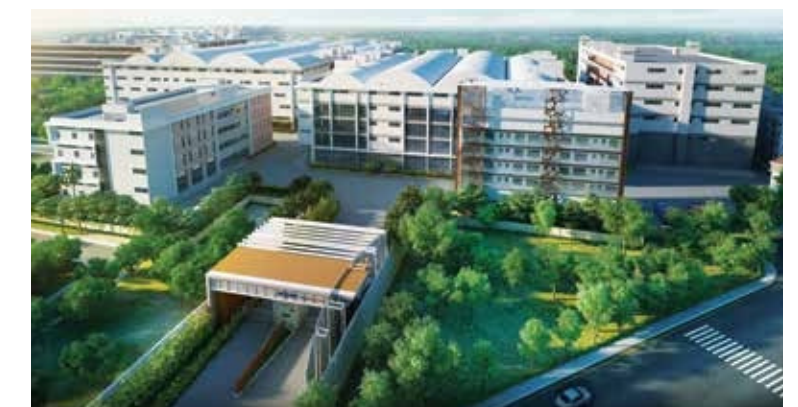
SRIJAN INDUSTRIAL LOGISTIC PARK on NH 6
